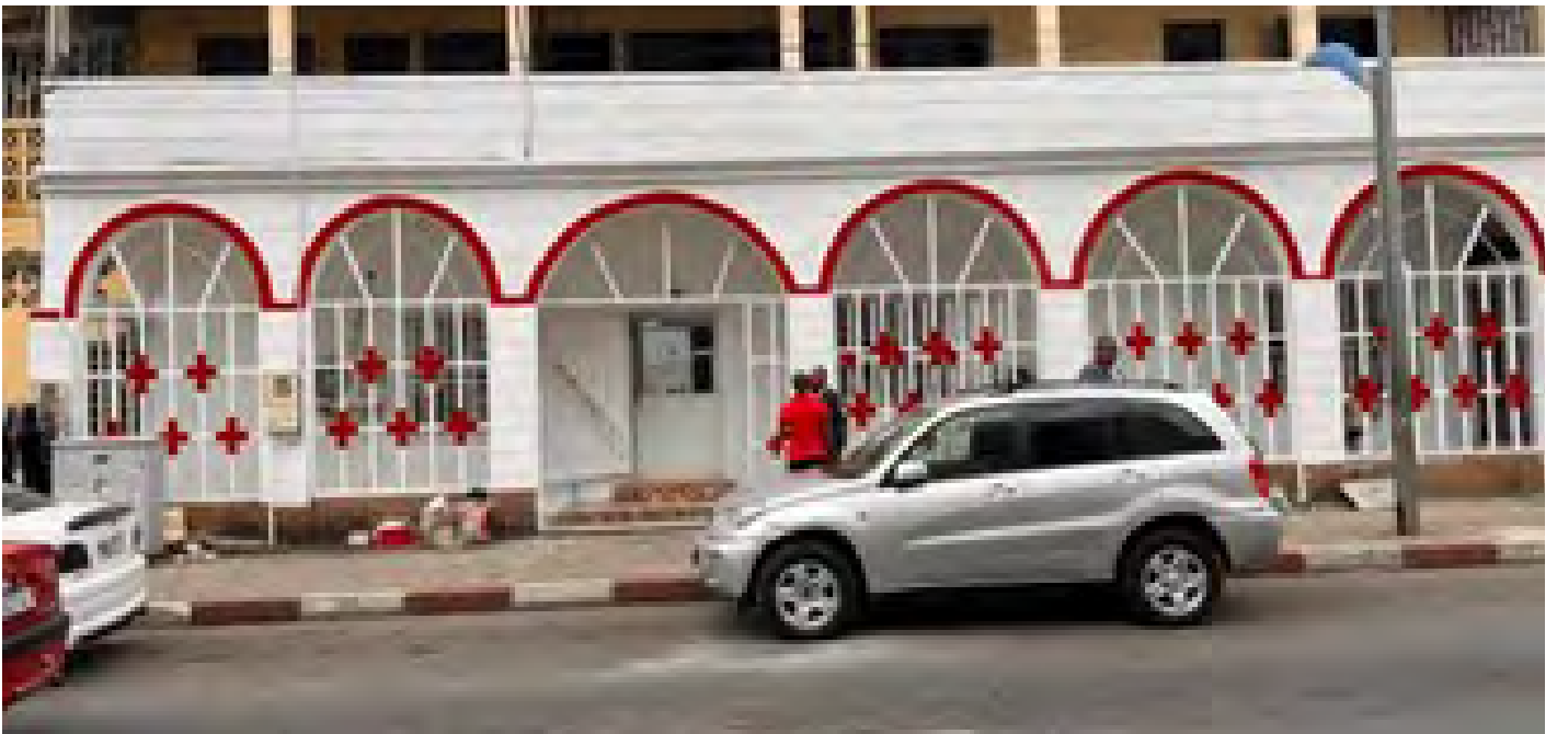
With the IFRC capacity building fund, the National Society carried out the rehabilitation of the headquarter building. (Photo: Red Cross of Equatorial Guinea)
